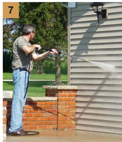
**7** When rinsing vertical surfaces, start at the top and work downward. Gravity will help the clean water flush away dirt, debris and detergent residue, in addition to preventing streaking.
