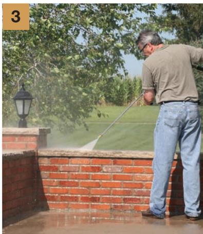
**3** Maintain a consistent distance between the nozzle and the cleaning surface.
