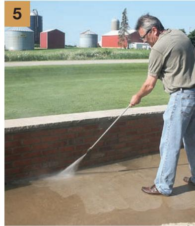
**5** Consider using brush attachments or a rotating nozzle to help remove stubborn dirt, grime and stains.
