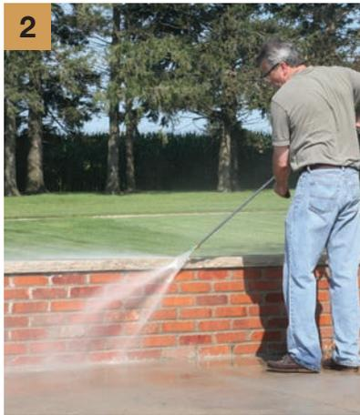
**2** Keep the nozzle in motion, spraying at a steady speed with long, even strokes to ensure uniform results.
