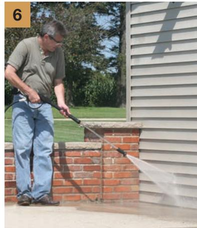
**6** To prevent streaks on vertical surfaces, such as fencing and house siding, always begin pressure washing or applying detergent at the bottom of the surface, then work upward.
