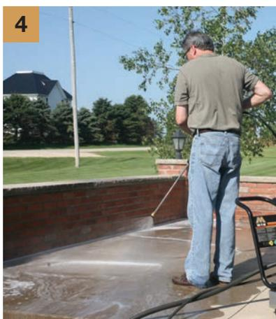
**4** When cleaning heavily soiled or stained surfaces, use cleaning detergents formulated for pressure washers. Be sure to NEVER use caustic cleaning agents.
